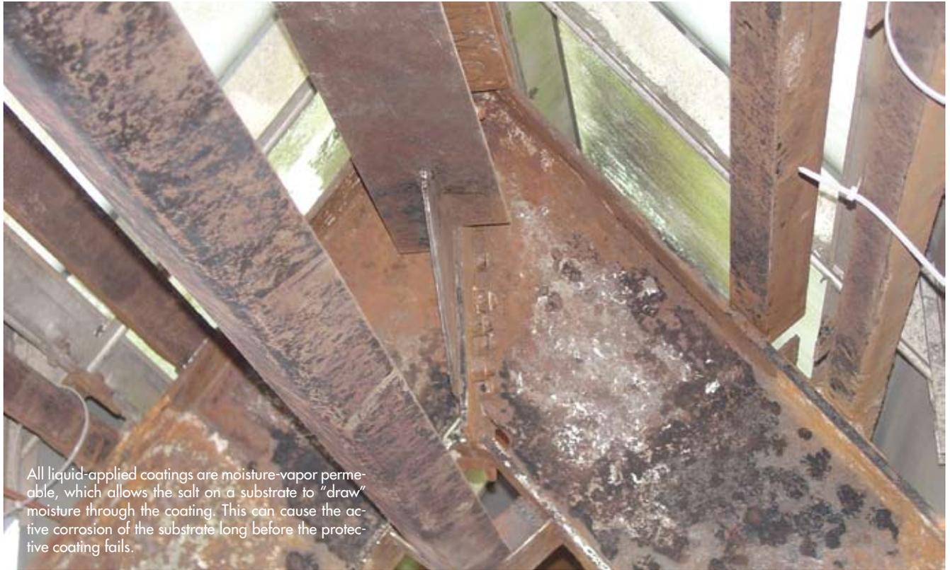
All liquid-applied coatings are moisture-vapor permeable, which allows the salt on a substrate to "draw" moisture through the coating. This can cause the active corrosion of the substrate long before the protective coating fails.
