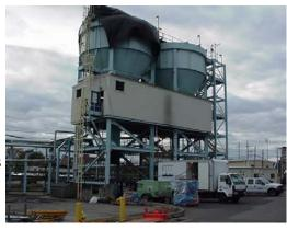
The application procedure called for abrasive blasting of the steel bin interiors to remove the epoxy system. This proved very difficult and air chipper / hammers had to be used to initially remove the 2-coats of flake filled epoxy. The area was then re-blasted to remove the corrosion and provide for a 3-4 mil profile. This was a compete confined space application so all the appropriate OSHA PPE was required.
