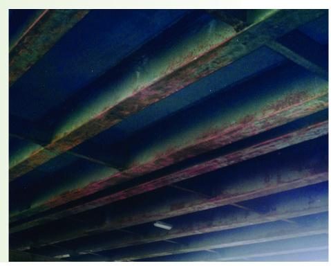
Fig. 1: Deicing salts have run down an open joint on the I-80 bridge, causing corrosion.
