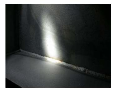
On April 2<sup>nd</sup>, those areas that turned after 2 vapor blastings with HoldTight102 were sanded with 80 grit paper to remove the flash rust. Hand repaired surfaces of the vapor trailer were then coated on April 3<sup>th</sup>.
