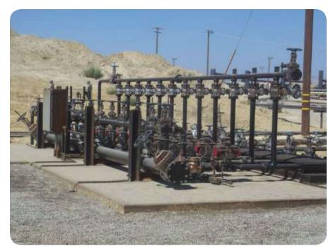
FIGURE 1 Steam injection platform.
