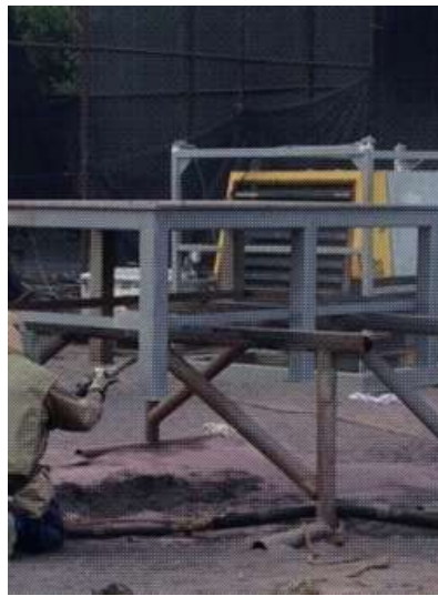
Photo # 17 (Finish Blasting)
