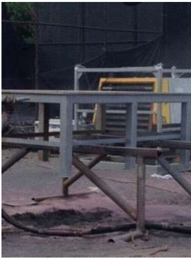
Photo # 16 (Finish Blasting)
