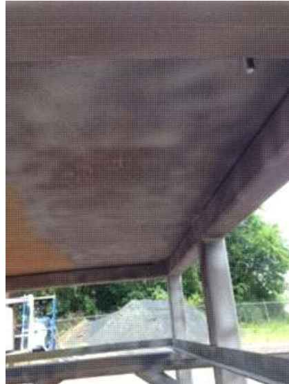
Photo # 13 (Rough Blasting)
