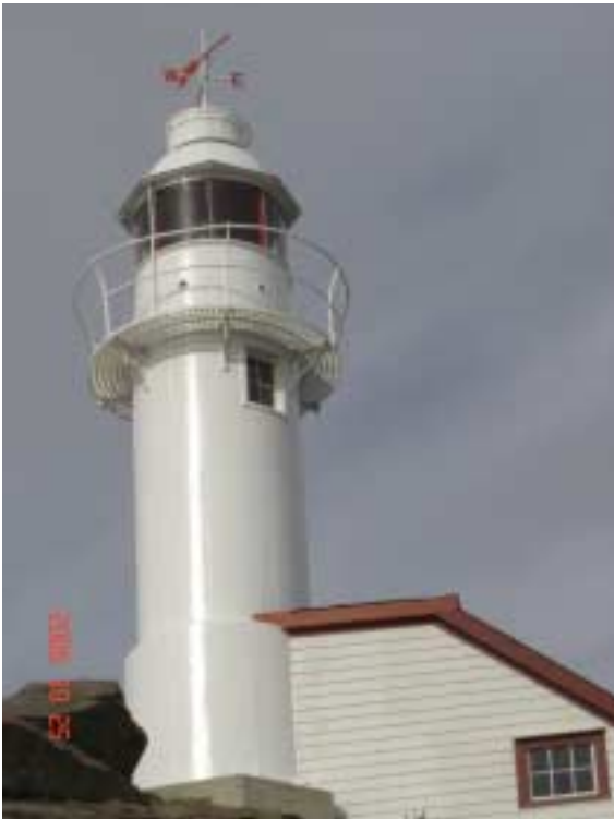
Photo #1: Lobster Cove Head Light Tower, est. 1897, cast iron tower. Rocky Harbour, NL.
