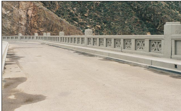
Deteriorated concrete curbs have been chiseled and cut out before repair, cleaning, and coating.
