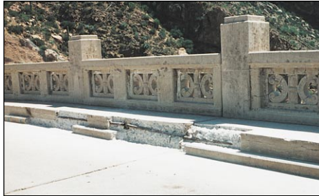
Deteriorated concrete curbs have been chiseled and cut out before repair, cleaning, and coating.
