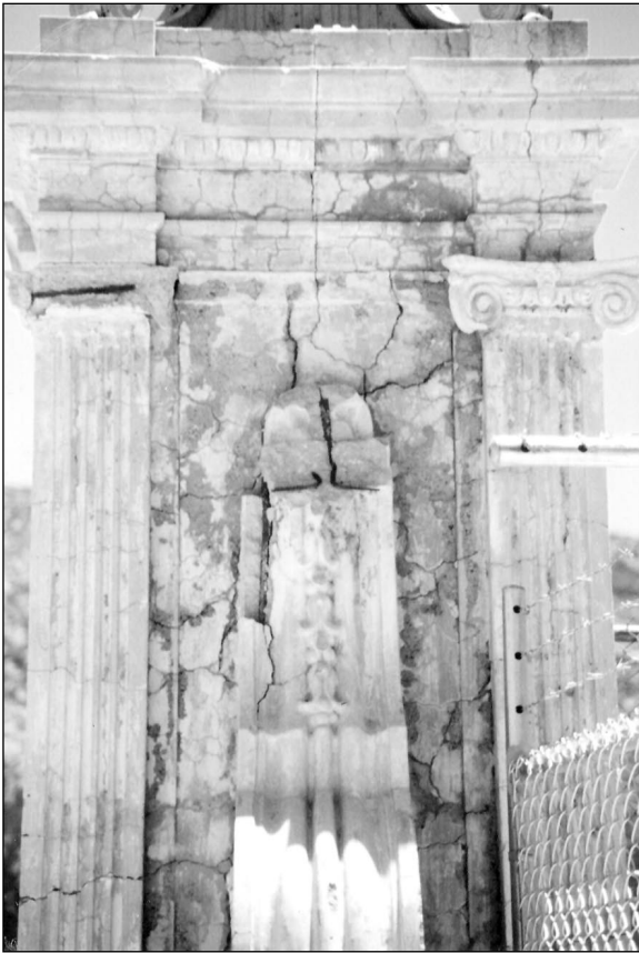
Above: The pylon, with coating intact, four years after repairing, removing soluble salts, and coating
