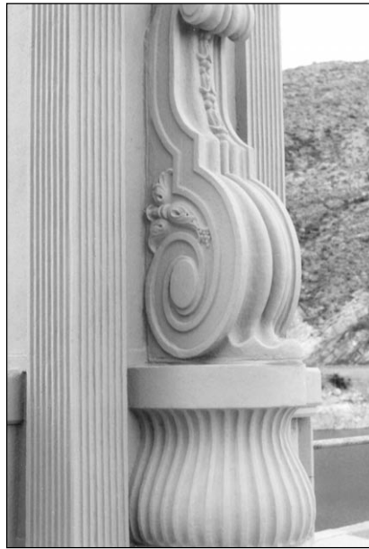
Above: The pylon, with coating intact, four years after repairing, removing soluble salts, and coating
