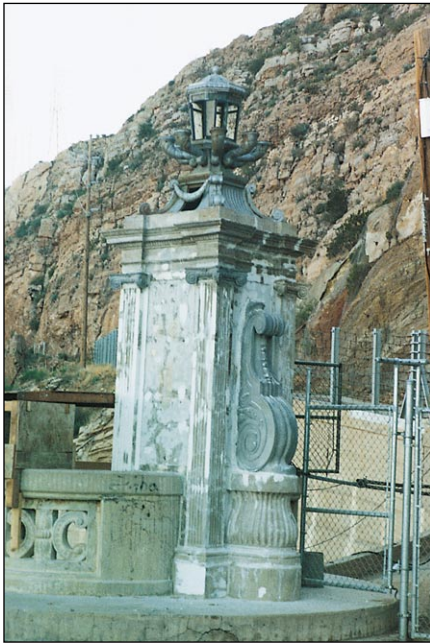
Pylon with plaque before any repairs were undertaken
