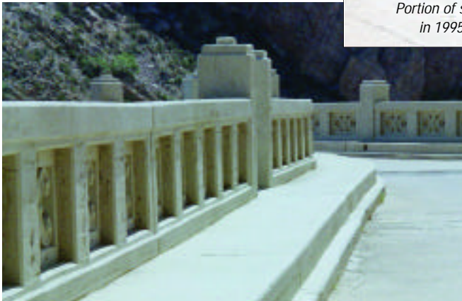
Curb and walkway on both sides of road 9 years after rehab
